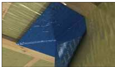
DAFA external corner on ceiling.
