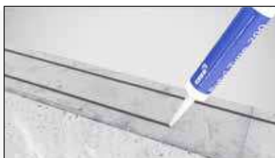
Sealing against plinth / foundation.
