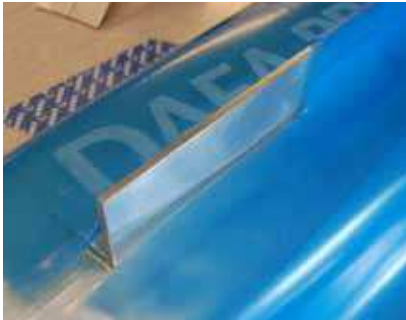
Sealing for breaks in the vapour barrier.
