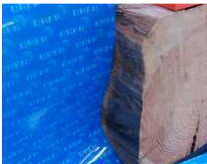
Sealing around difficult surfaces, e.g. old structural floor.
