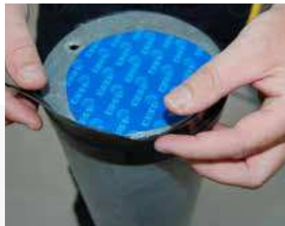
Remove the other half of the backing sheet and tilt DMS up towards the foil.
