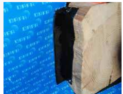
Fold out DMS and fasten it to the foil.
